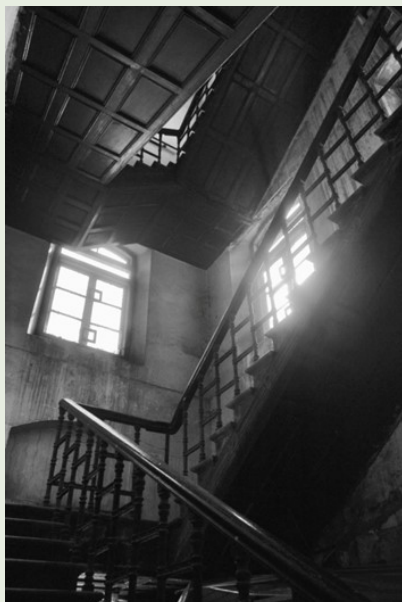
Open well stair
